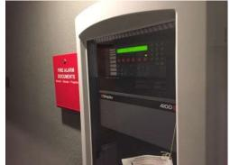
**Description:** There is a fire controller/communicator in the office adjacent to the entry foyer. Throughout the building there are smoke and heat detectors, pull stations and water-flow sensors at the fire sprinkler system.
