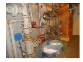
**Description:** The fire sprinkler system with associated valves and piping.
