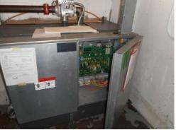
**Description:** Elevator control systems for the two passenger elevators.
