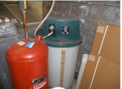
**Description:** There are various valves and expansion tanks that are used for the domestic hot water, heat and snowmelt systems.
