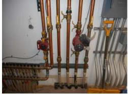
**Description:** There are various commercial heating and hot water circulation pumps and motors.
