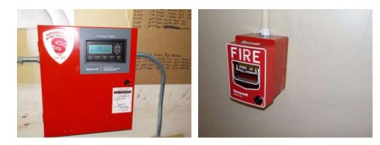
**Description:** There is a fire controller/communicator and fire alarm annunciator. Throughout the building there are smoke detectors and pull stations.
