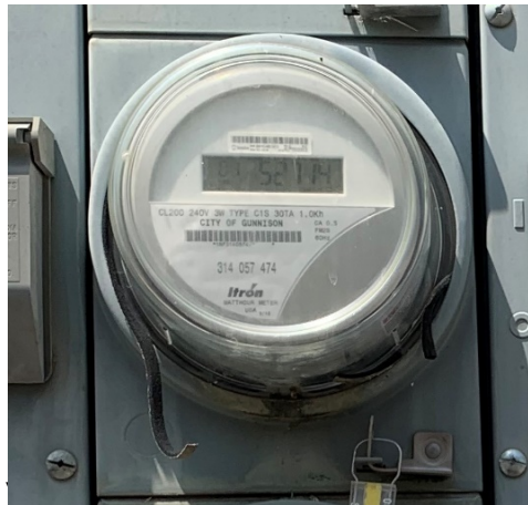
Aging Meter with Deteriorating gasket
