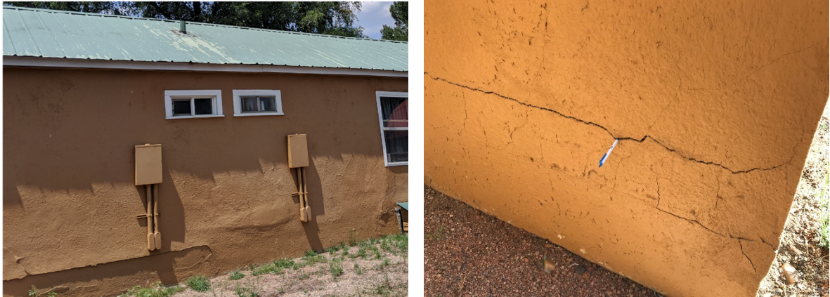
Cracked stucco at crawlspace and window sill or foundation
