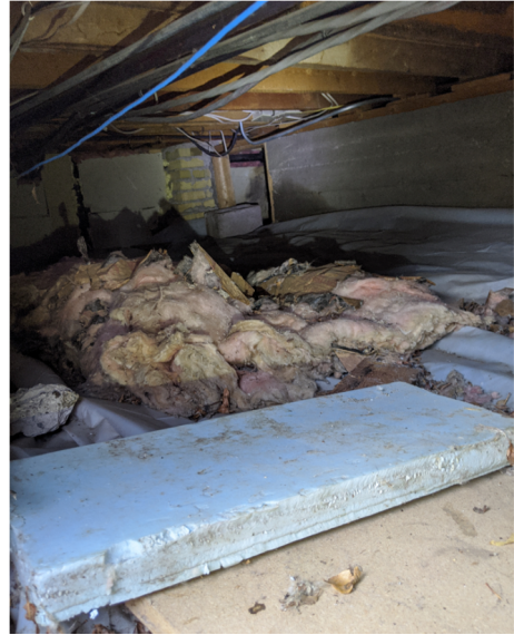
Damaged/uneven insulation.
