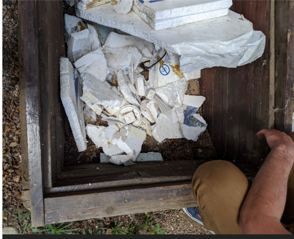
Trash blocking crawlspace access.
