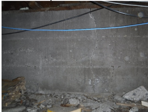
Foundation wall - Cracked but in reasonably good condition
