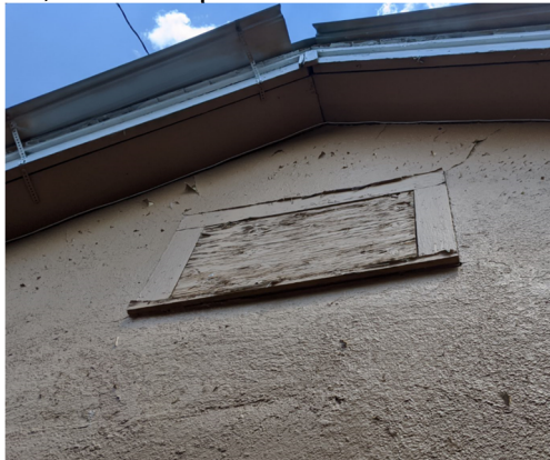
Attic vent blocked off on Building 2.
