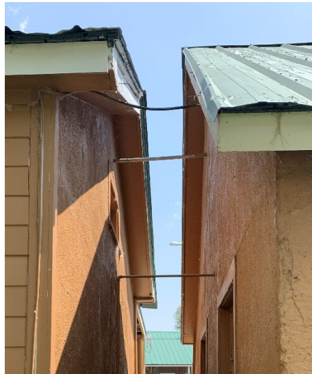
Conduit and Cable Between Buildings
