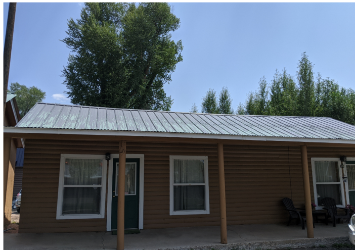
Sagging roof and peeling paint on Building 1.
