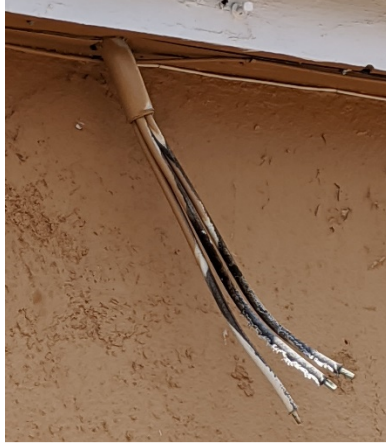
Example of Cut Feeders
