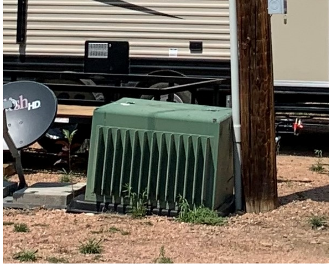
East Transformer Settling
