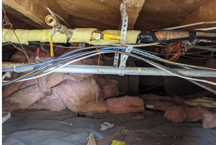
General disarray of utilities in crawlspace. Note the incomplete piping insulation, lack of labeling, and exposed piping end at branch secured only by valve closure.
