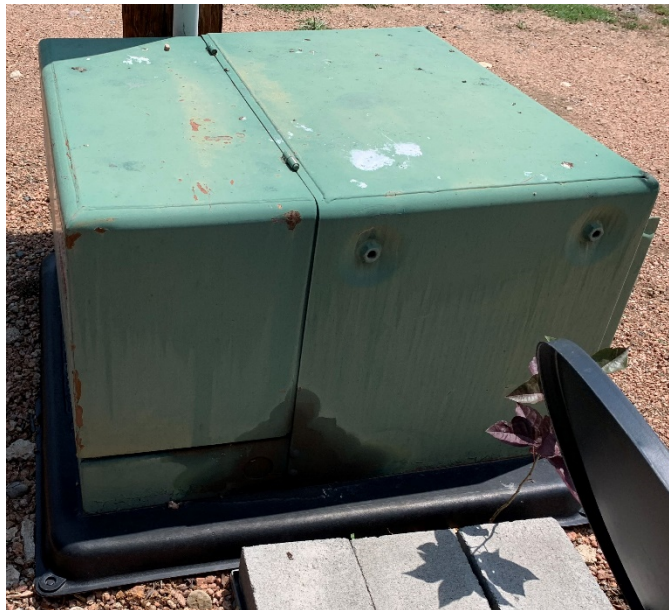
East Transformer Water Ingress
