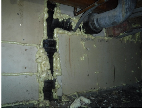
Sewer pipe running through fire wall.
