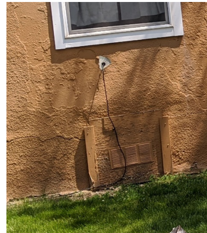
Improper Cable Installation
