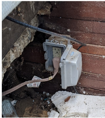
Example of Improper Use of Exterior Receptacle (Note that the cord is also not rated for outdoor use)
