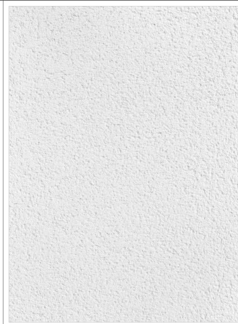
1 3-PART STUCCO W/ ELASTOMERIC PAINTED FINISH COAT; BENJAMIN MOORE 'SIMPLY WHITE'
