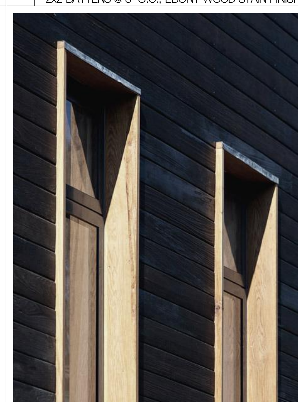
5 1 1/2" NARROW PROFILE SOLID WOOD TRIM ELEMENTS; NATURAL CLEAR WOOD SEALER
